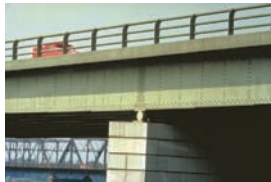
Bridge with roller support (see 1.1, 1.2)
